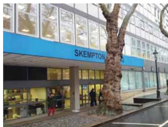
Centre for Transport Studies の建物 Skempton Building (Imperial College London)
