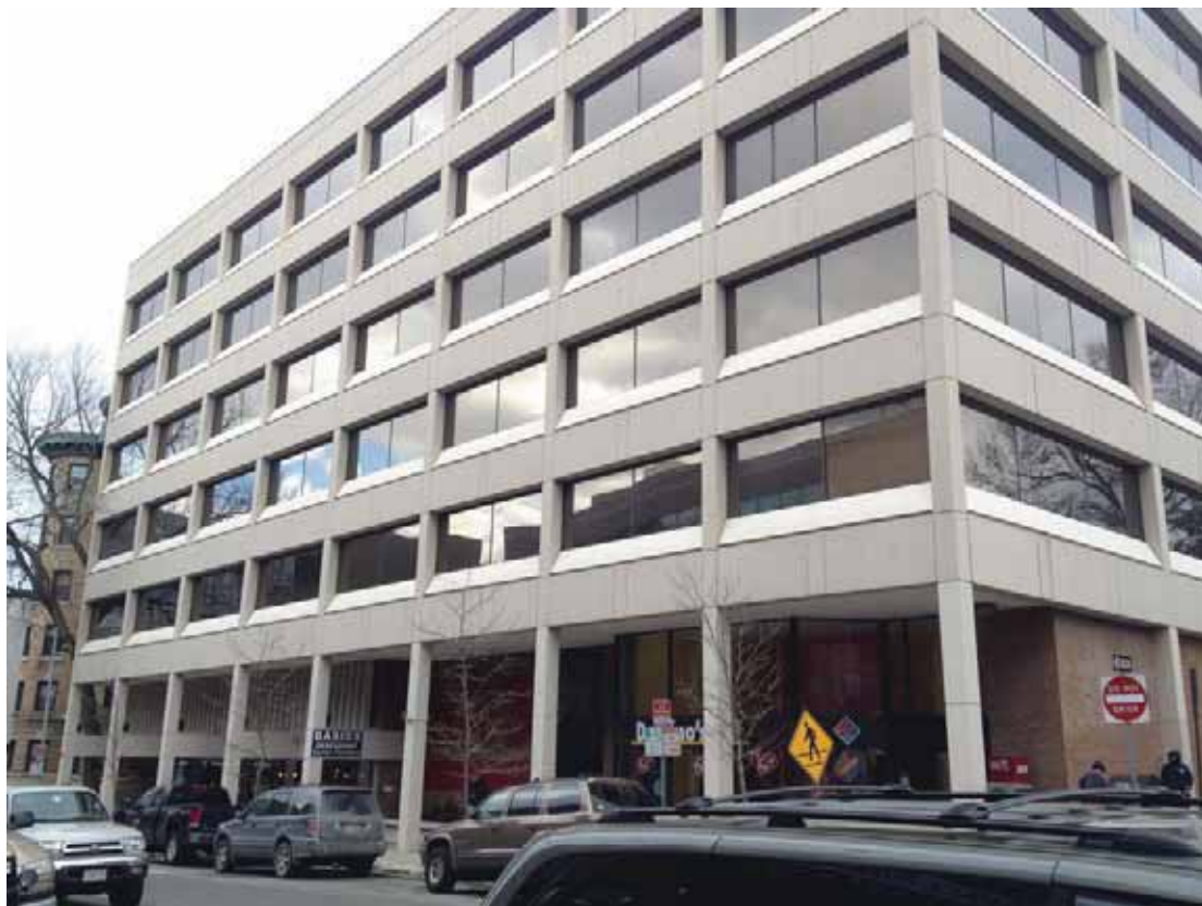
Joint Center of Housing Studies の入るビル
